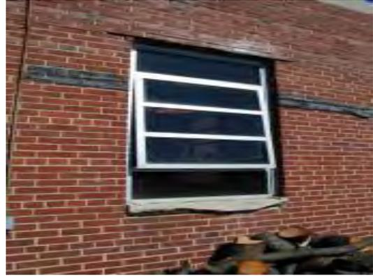
Un-caulked/un-sealed exterior wall penetrations and damaged window sills
