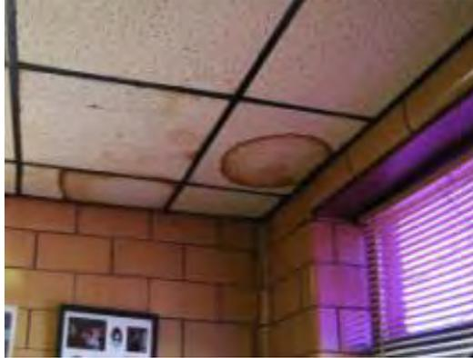
Signs of standing water/pooling, standing water 4 inches high, and signs of water damage on interior finishes.
