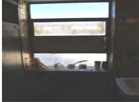
Air-leakage at sleeved window/wall air-conditioning units in outdated single glazed windows units
