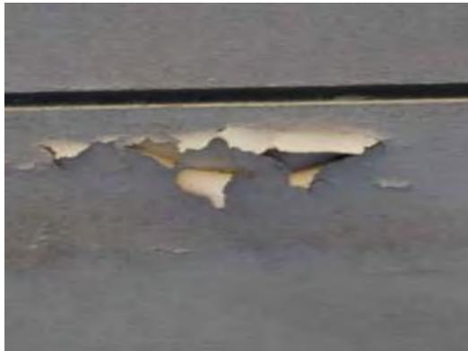
Deteriorating interior and exterior wall finishes due to water/moisture presence inside the wall cavity
