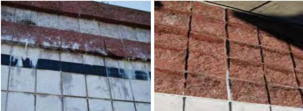
Signs (mostly efflorescence) of uncontrolled roof water runoff on walls due to missing/defective roof flashing
