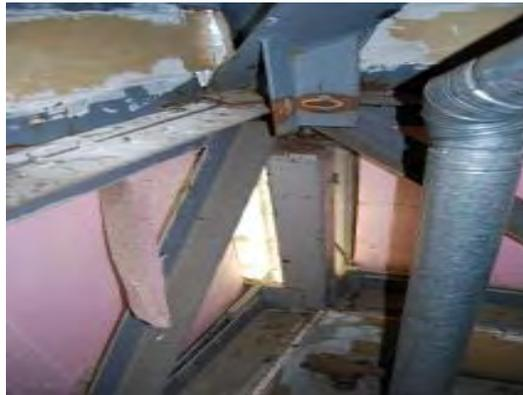
Uneven, ineffective and inconsistent attic and roof insulation found
