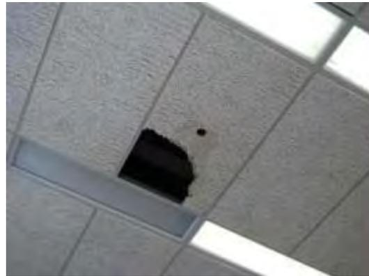
Signs of water damage on ceiling tiles due to significant roof leaks in two areas of the building.
