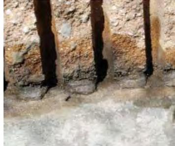
Deteriorating exterior and interior wall finishes due to water and moisture presence inside the wall cavity
