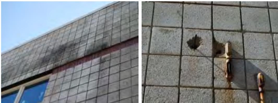
Mold and water stains on brick and masonry walls indicate possible moisture presence within the wall cavity.
