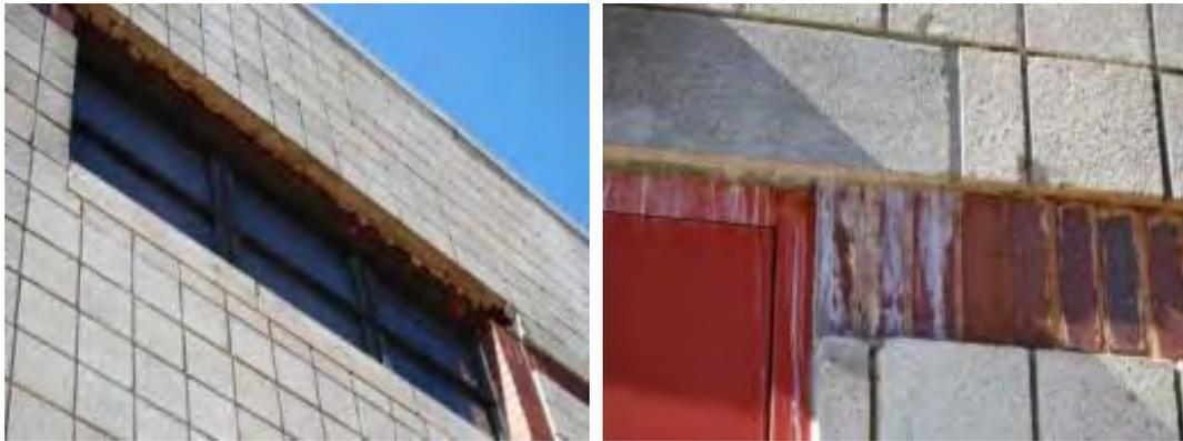
Rusted/deteriorated steel lintel and efflorescence on brick and masonry walls indicate moisture presence within the wall cavity
