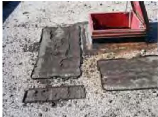
Glass, rocks or other sharp objects on roof surface and delaminating roof membrane patches
