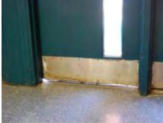
Damaged and aged door frame with missing weather- stripping.
