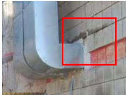
Signs of water damage at perimeter walls
